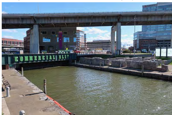
Above: Modern image of the Commercial Slip in Buffalo, NY.
