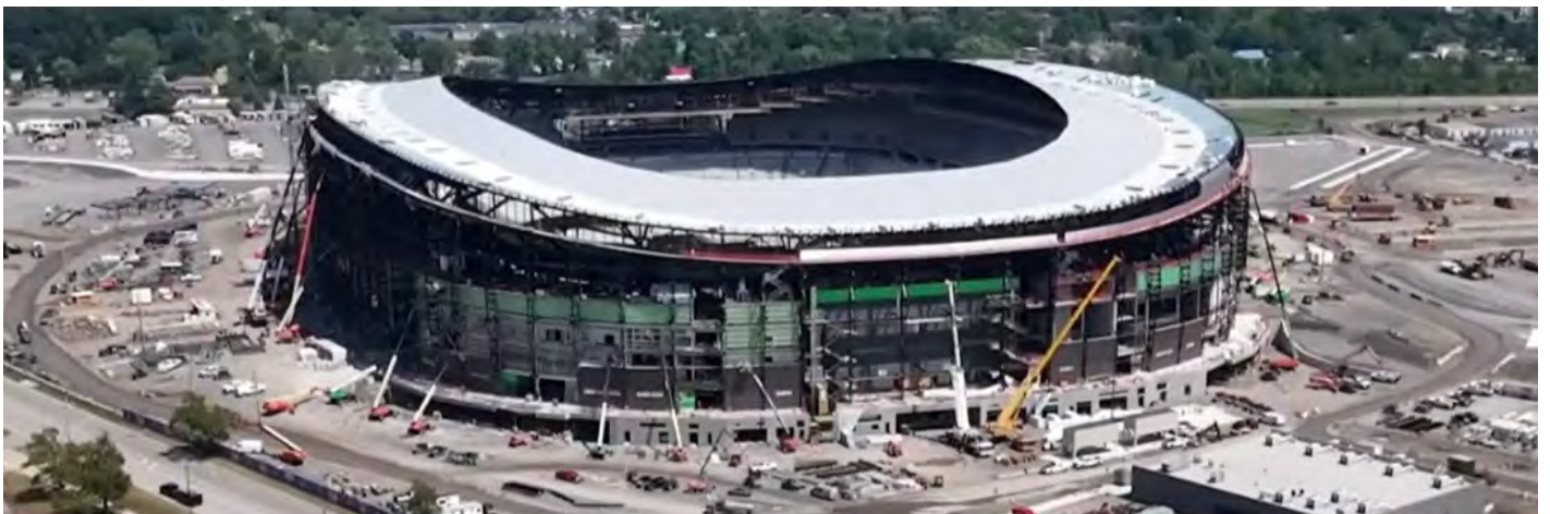
Construction progress photo of the new Buffalo Bills Stadium, August 3, 2025 (Photo from SportsRender.com, by Arlind)
