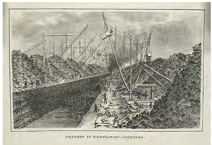
Original excavation of Erie Canal Locks at Lockport, NY
