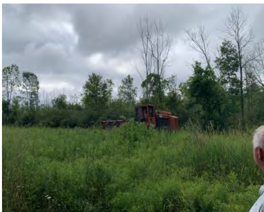
Construction commences on July 31, 2024.
